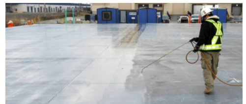
CURING OF CONCRETE
