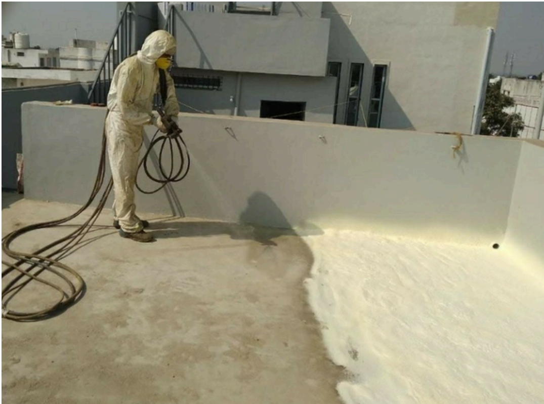
The application of polyurethane foam insulation.
