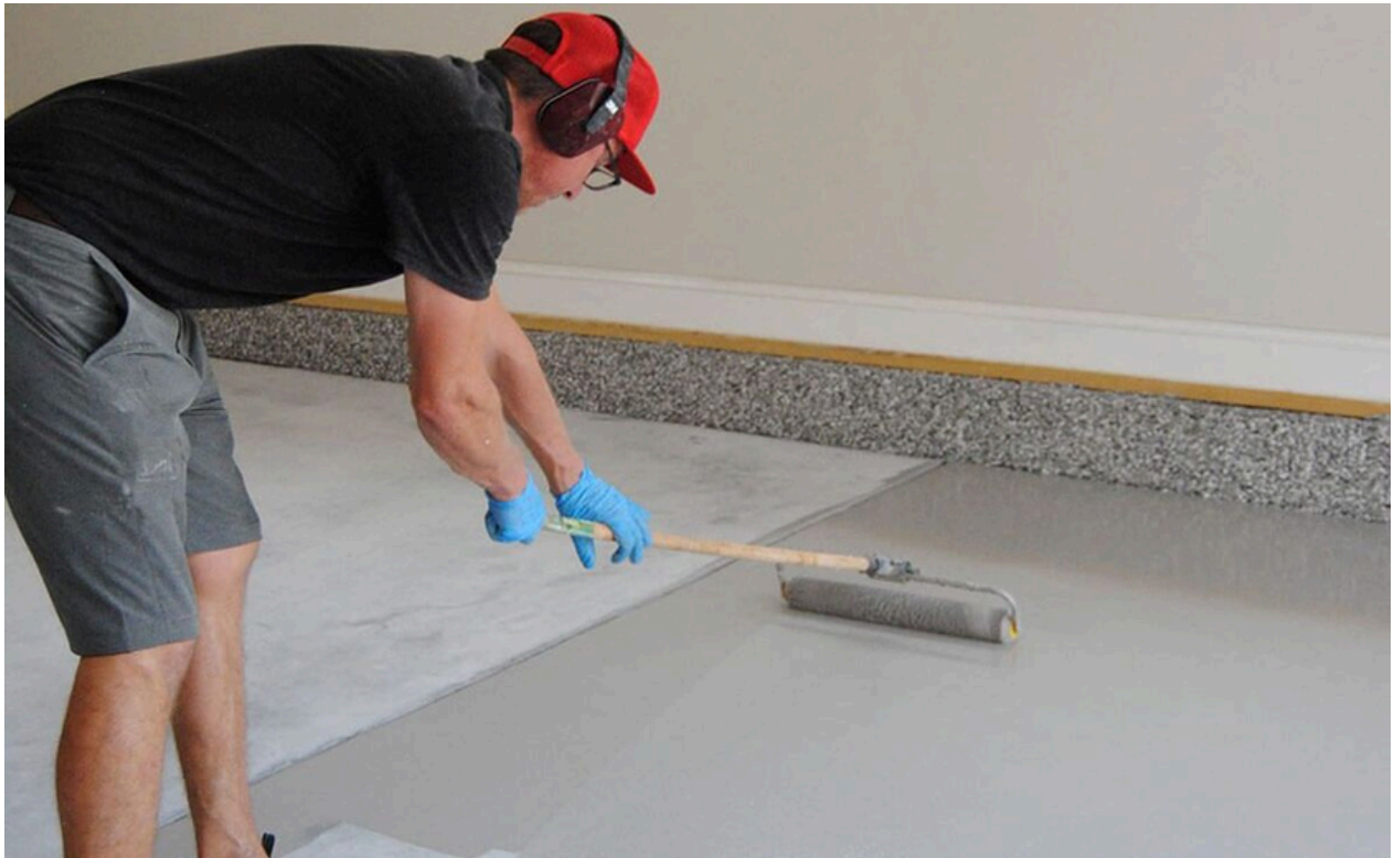
The application of epoxy painting works on the Outdoor Floor.
